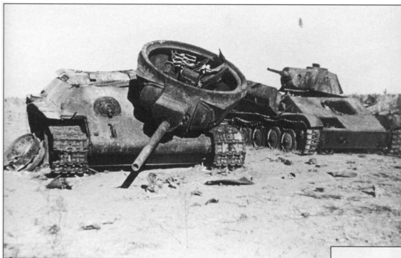
Two more Soviet tanks demolished by German anti-tank rounds. At left is a T-34 with a torn-off turret; at right is a T-70 whose superstructure is ruptured. In those days Soviet tank units had limited chances for success due to the lack of radio, good tactics and knowledge of co-operation with other sorts of weapons — they could only charge straight into enemy guns until the last tank was
