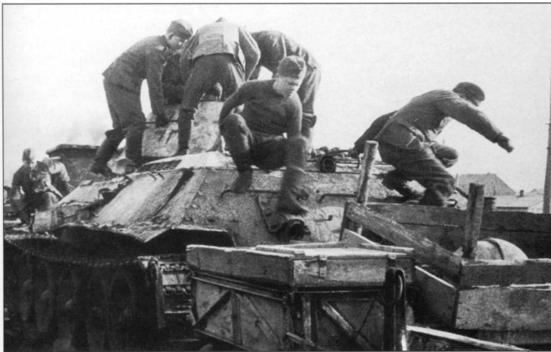
A captured T-34 tank is ready for transport by rail to the rear. The tank, which is from a pre-winter 1941 series, is covered with a thin coat of whitewash and has the German black national cross on the turret. The soldiers of the Panzerwaffe greatly appreciated the T-34, mainly due to its simplicity and good maneuverability. Therefore, this tank saw service in many German armored and anti-tank units.
