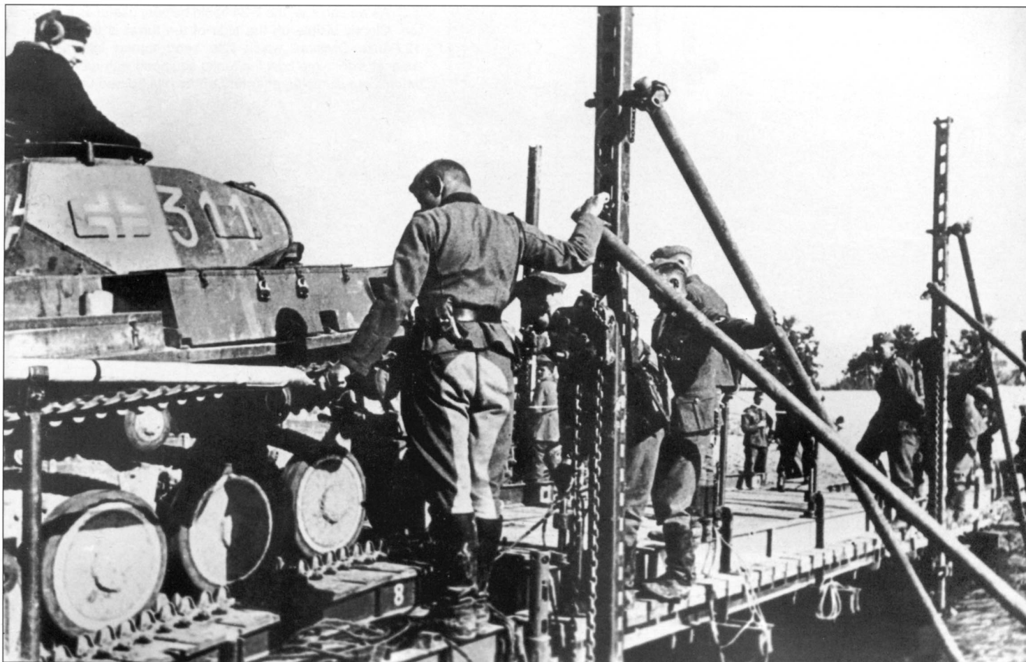
A Pz.Kpfw. II crosses the Dniepr river courtesy of a light bridge built by an engineer battalion in July 1941. The material under the tank tracks is a piece of light assault bridge used by motorized engineer troops in Panzer divisions, usually transported on the Sd.Kfz. 251/7. Of special interest are the markings on the turret, composed of white national cross and the yellow tactical number "311" on all three sides. The tank probably belonged to Pz.Abt.(F) 100 or 101.
